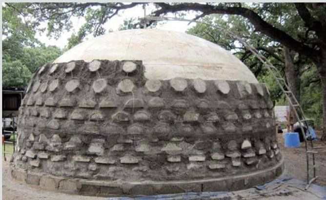
Dome is shown here partially completed with scaffold and air form inflated.
