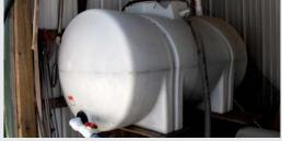
A 350-gal. tank is also used to collect rainwater from barn roof and serves as a backup.
