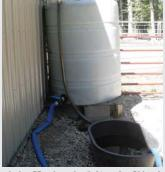
Amy Childs's rainwater collection system includes 55-gal. tanks (left) and a 500-gal. tank that collects rainwater from her barn's roof.
