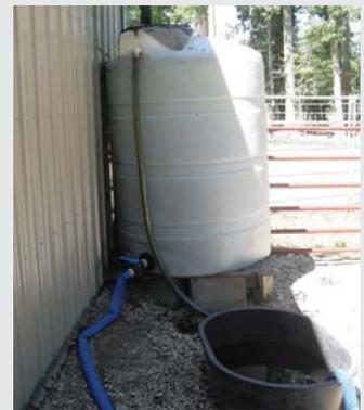
Amy Childs's rainwater collection system includes 55-gal. tanks (left) and a 500-gal. tank that collects rainwater from her barn's roof.
