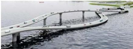
Computer-generated photo shows how innovative design automatically switches cars from one side of the road to the other.
