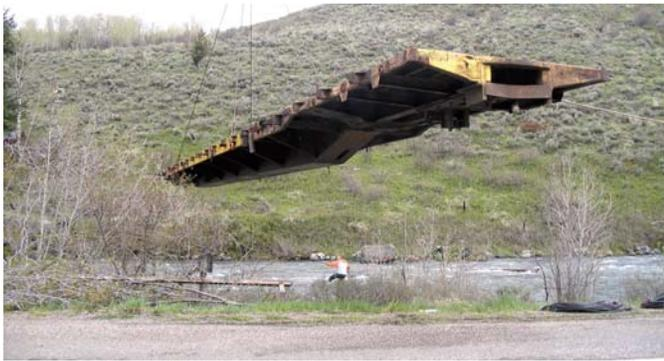
Recycled flatbed railroad cars can be converted into a wide variety of bridge sizes and styles, says Paragon Bridge Works.
