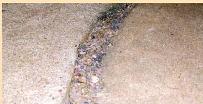
Cracks in asphalt driveways and concrete floors can be filled with expandable spray insulating foam topped with crack filler and grit, says Roger Meihak.
