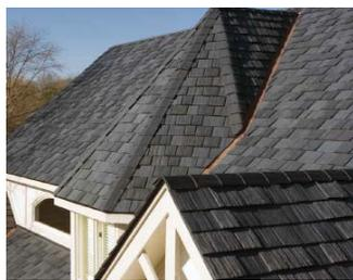
Made from recycled rubber tires, rubber “shingles” are a good alternative to expensive slate or shake roofing, says the manufacturer.
