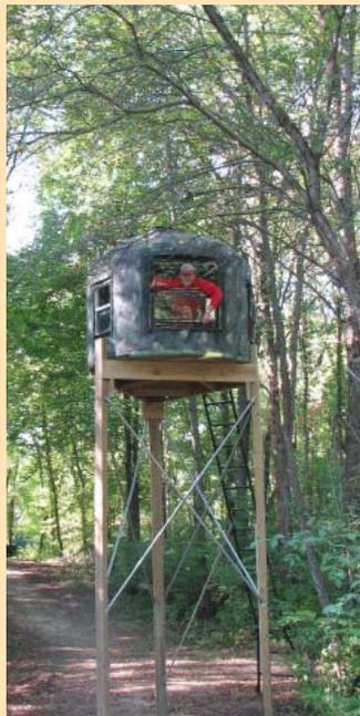
John Siefker turned a 1,200-gal. poly tank into this low-cost deer blind. It sets 14 ft. high on top of a tripod wooden frame.
