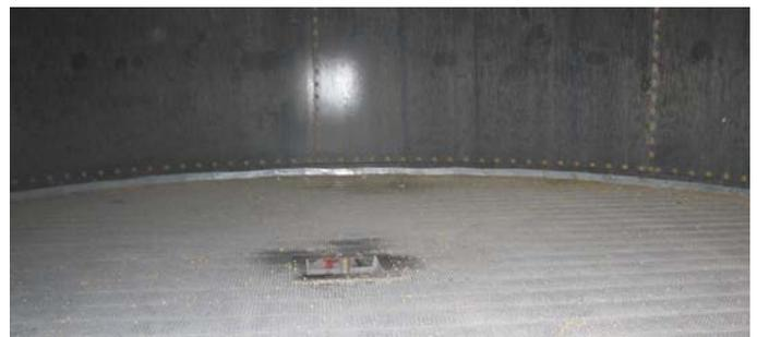
A 5 hp, 20-in. fan pulls air down through drying floor in the 20 by 32-ft. structure.
