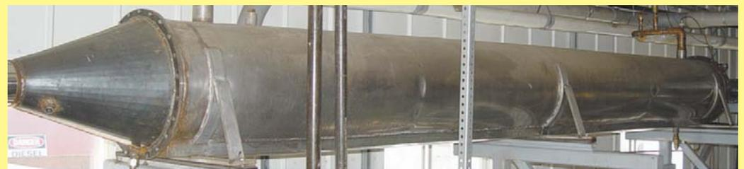
Heat exchanger uses diesel engine exhaust to heat water that runs through shop's radiant floor heating system.
