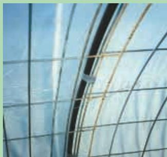
Panels are wired together at 2-ft. intervals where they meet. Wire ties are covered with duct tape to keep from tearing the plastic.
