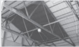
too often but it's annoying when it does. To eliminate the problem with a minimum amount of work, I stretched a sheet of lightweight plastic tarp under the rafters in such a way that water dripping through is directed over to the edge of the wall."
