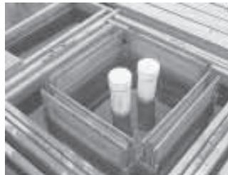
Kelsey Hydro System intake pipes and filter trap (left). Intake tank catches water coming off dam.
