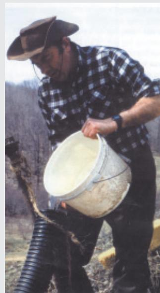
To keep his farm pond from overflowing, Art Briggs-Jude used a 50-ft. section of flexible 4-in. drain pipe as a giant siphon. He sealed off the bottom, left, and filled the pipe from the top using a 5-gal. bucket.
