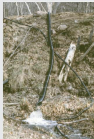
Water swooshed out lower end of pipe plug right through the pipe and out the other end as well. The siphon quickly lowered the water to a safe level.
