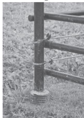
**Metal corner post is set inside a concrete-filled piece of flexible plastic pipe.**
