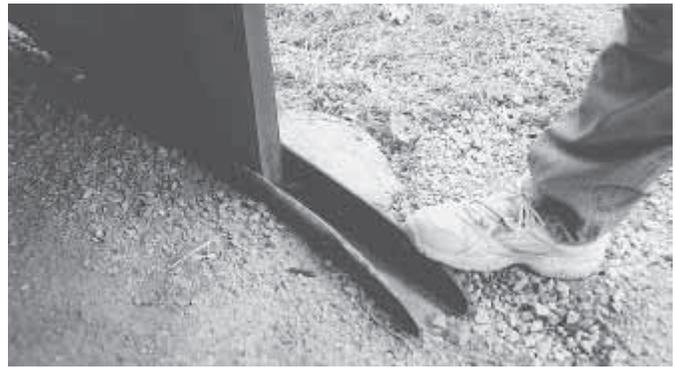
Channel guide is about 3 ft. wide at center of door opening. It prevents damage to sliding doors in strong winds.
