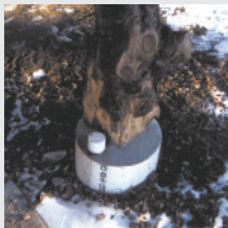
Every few months Jennings pours oil in through a concrete cap to soak the post.
