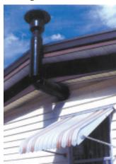
Black stove pipe is designed to cool the home. A venturi pipe at the top draws warm air out of home and cool air up from under the house
