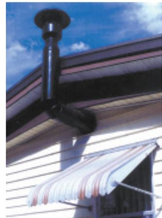
Black stove pipe is designed to cool the home. A venturi pipe at the top draws warm air out of home and cool air up from under the house.
