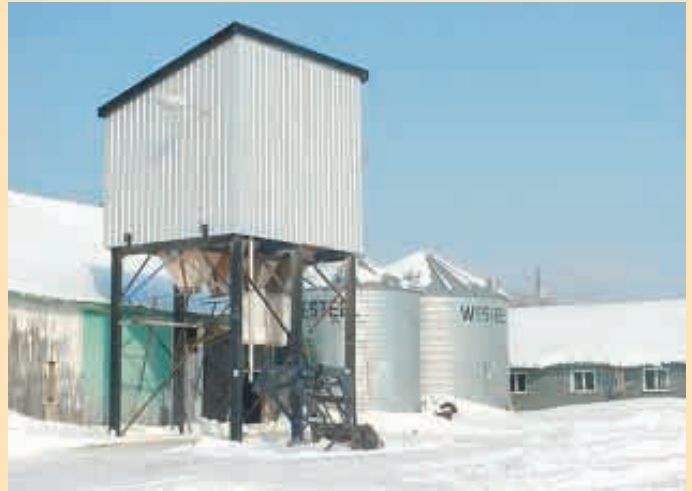
David Carrier built four bins high off the ground so he could drive under for a quick fill.
