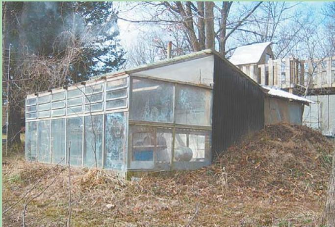
Greenhouse is built into side of hill, with heat from the ground keeping the greenhouse warm. A cement mixer drum is buried in the hill side behind it.
