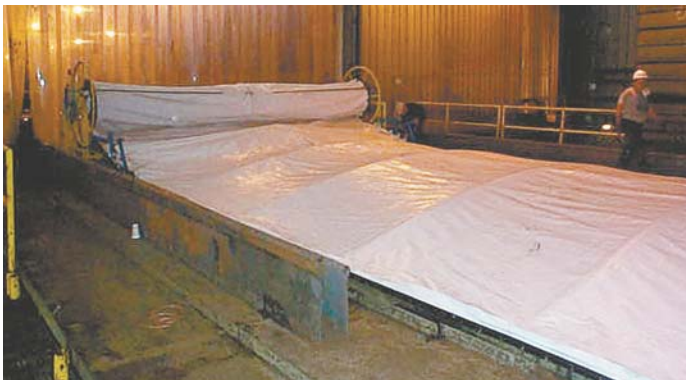
Retractable cover is 20 ft. wide and half a mile long and covers a 10-ft. deep trench that holds manure.
