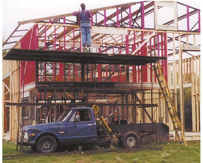
Pickup-mounted pin and socket pipe system lets Montalbano add scaffolding as needed.
