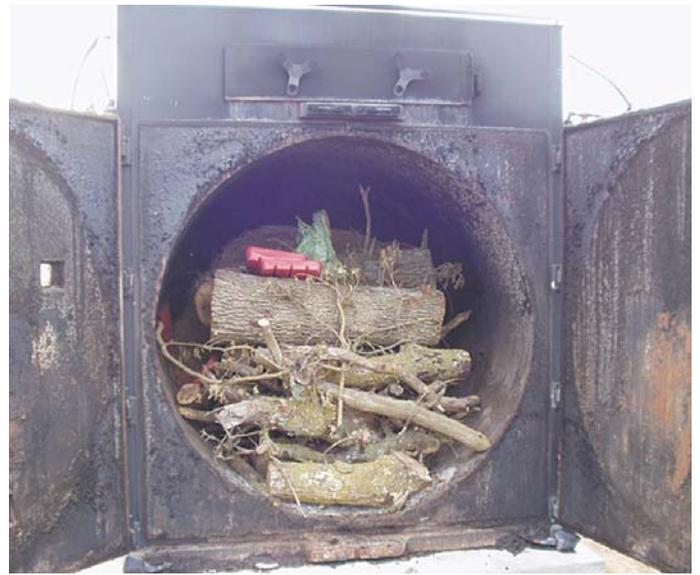
System includes a 10 by 8-ft. furnace with a 7-ft. door to load round bales, a 4,000-gal. water tank, water lines, and radiators .
