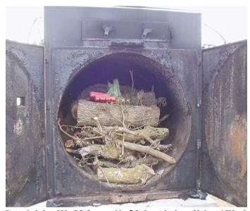
System includes a 10 by 8-ft. furnace with a 7-ft. door to load round bales, a 4,000-gal water tank, water lines, and radiators .
