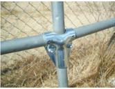
This clamp was used to repair a pipe joint that had rusted away.
