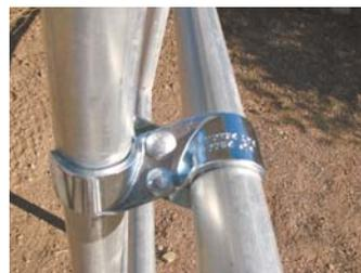
**Pole clamp has a figure-8 twist that allows the connection of vertical and horizontal pipes.**
