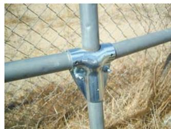
**This clamp was used to repair a pipe joint that had rusted away.**
