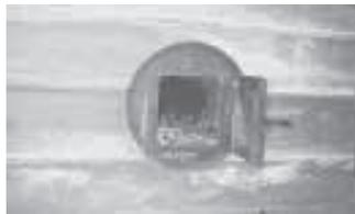
**A 55-gal. barrel stove mounts in an outside wall.**
