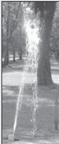
As hole is dug, water and dirt shoot out, carried by air exiting tool.
