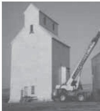
Attached grain bin was moved away before work was begun.
