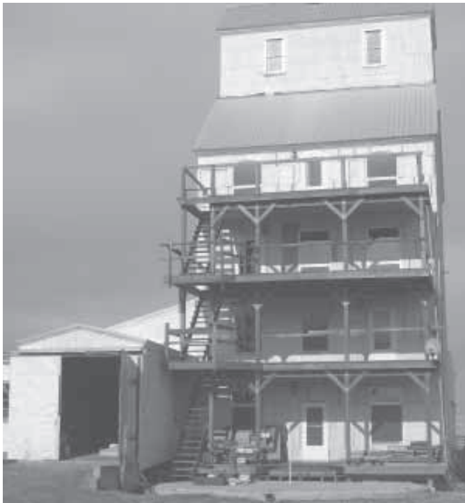
A remodeled country elevator serves as a unique retirement home for Jill Baumlér and her husband, Bob Mannisto. They live on the top four stories.
