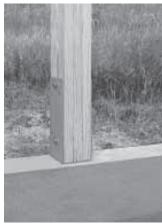
To install post, slip Perma Column bracket with its four rebar studs into the wet concrete and let it harden before inserting the nost.
