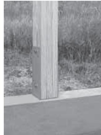
To install post, slip Perma Column bracket with its four rebar studs into the wet concrete and let it harden before inserting the post.
