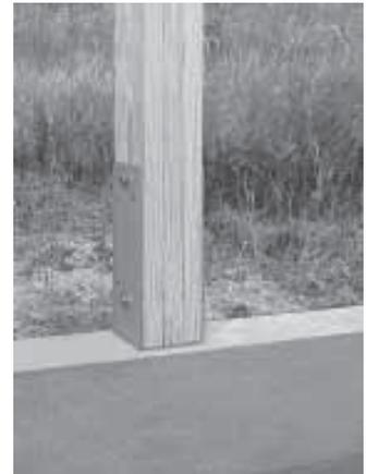
To install post, slip Perma Column bracket with its four rebar studs into the wet concrete and let it harden before inserting the post.
