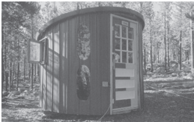
Jon Bell used a satellite dish for a roof and vertically positioned roofing tin to make the walls on this storage shed. Note elliptical windows cut into the tin walls.
