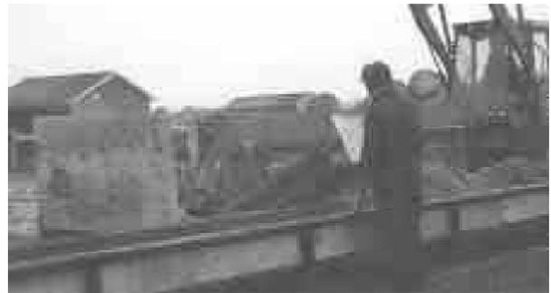
The Woywitkas unbolted the paddles from the spreader beaters and bolted on a two-piece rubber belt conveyor below and behind the back of spreader.
