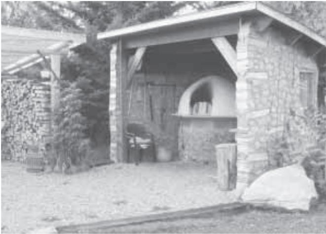
"Outdoor kitchen" is built from cordwood stacked and mortared together like bricks.
