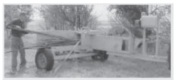
Casper Holter stripped the tieing assembly from a wire-tie Case baler, leaving only the plunger. He piles boards up on pickup table, then feeds them one at a time into plunger.
