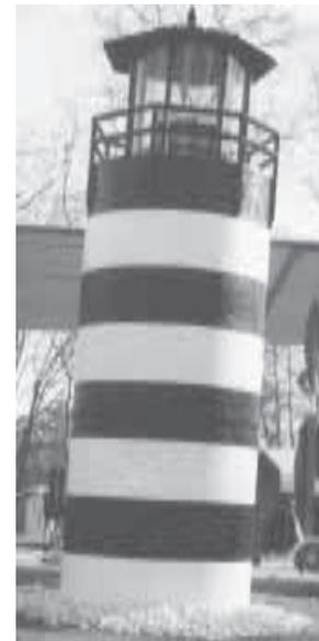
Lighthouse was built by standing an old fuel tank on end and then building a light cage on top.
