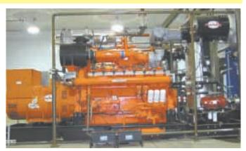
Heat recovery unit, right, produces hot water using "waste heat" off this stationary diesel-powered generator
