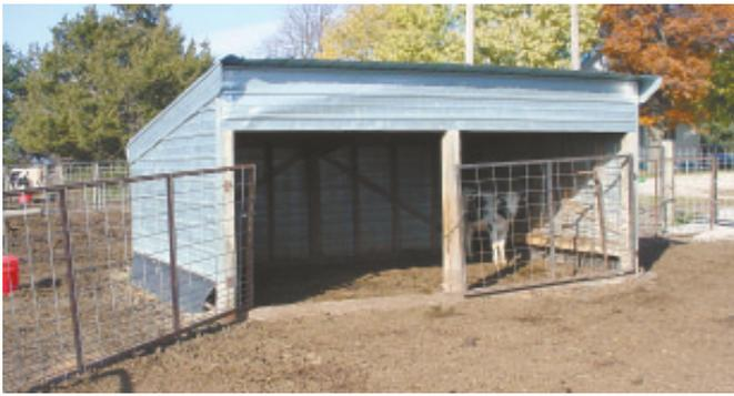
Buildings mount on runners so they can be easily moved. A strip of rubber belting runs across ends of shed. As building is towed to a new location, the belt helps the building slide up and over manure.
