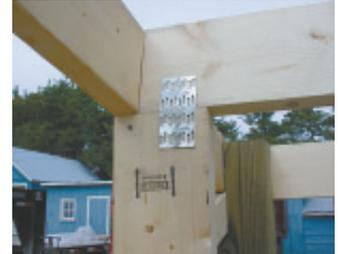
Schweppe uses 6 by 6 treated posts on building's corners for maximum strength. They're notched at top (left) to accept 2 by 6's, which hold the sides up and also support the rafters. Metal connector plates that hammer in place are used to attach the 6 by 6 corner posts to runners.
