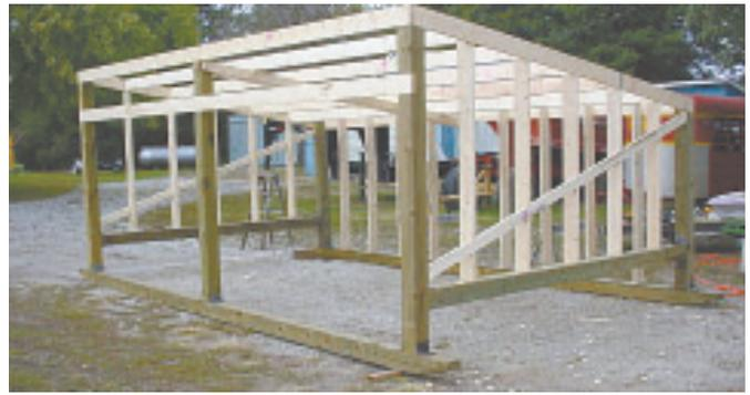
Framing is made from notched lumber for extra strength and to provide a smooth surface for applying metal siding.
