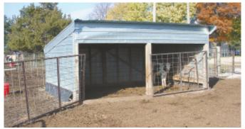
Buildings mount on runners so they can be easily moved. Astrip of rubber belting runs across ends of shed. As building is towed to a new location, the belt helps the building slide up and over manure.
