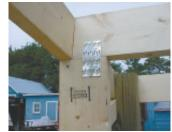
Schweppe uses 6 by 6 treated posts on building's corners formaximum strength. They're notched at top (left) to accept 2 by 6's, which hold the sides up and also support the rafters. Metal connector plates that hammer in place are used to attach the 6 by 6 corner posts to runners.
