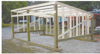
Framing is made from notched lumber for extra strength and to provide a smooth surface for applying metal siding.
