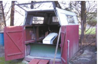
Ken Booth used the topper off a small Dodge pickup as a roof for a small shed.
