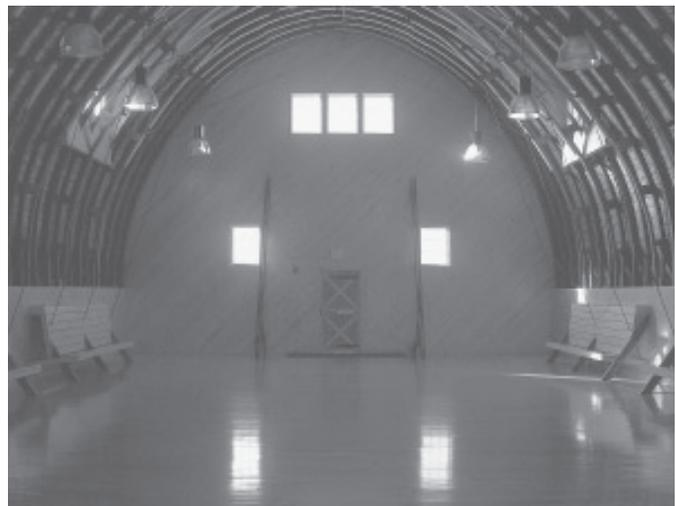
**Barn's floors were replaced and interior walls sided, except in the old haymow where the original bent wood rafters can be seen.**
