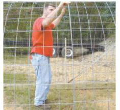
He bent a 16-ft. long cattle panel, placing the ends inside both boards. He stapled and nailed the panel to the wood and wired the panel to the T-posts. Then he installed a second panel, tying the ends of the two panels together.
