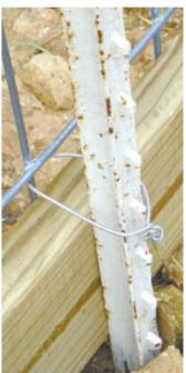
He started by pounding four T-posts into the ground, placed parallel to each other 84 in. apart (left). Then he placed a 16-ft. long, 2 by 8 wood board along each side.
