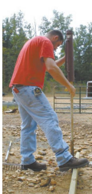
He started by pounding four T-posts into the ground, placed parallel to each other 84 in. apart (left). Then he placed a 16-ft. long, 2 by 8 wood board along each side.
