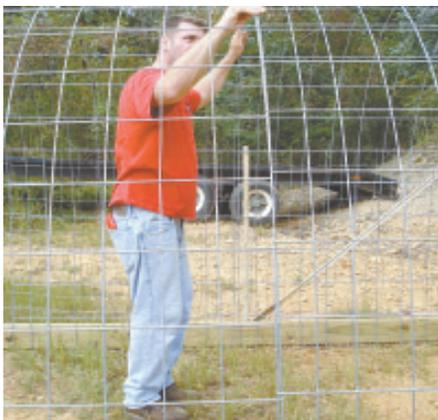
He bent a 16-ft. long cattle panel, placing the ends inside both boards. He stapled and nailed the panel to the wood and wired the panel to the T-posts. Then he installed a second panel, tying the ends of the two panels together.
