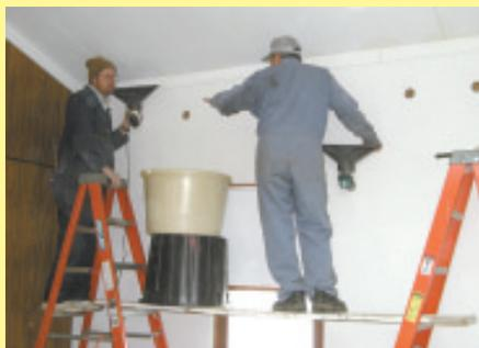
Roger Gutschmidt helped his church save on heating costs by "topping up" the building's existing insulation with Vermiculite. He drilled a series of holes in the walls and made funnels out of spray cones to blow the material in.
