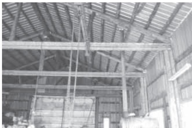
**Framework on Richard Stephens' 40 by 60-ft. shop is made from 14 and 26-ft. long sections of highway guard rails.**
