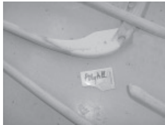
This broken piece of wood trim was repaired with PolyAll, which can be sanded down after drying.
