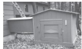
**"If there's ever a leak or something has to be replaced, I won't have to dig in the ground to get at it," says Ken Voigt, who ran the 1-in. water line from his pump house through an "insulated" bridge that's about 2 ft. off the ground.**
